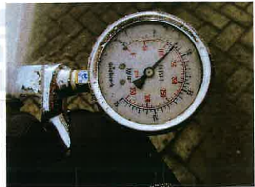
Percobaan operasional Hydrant
