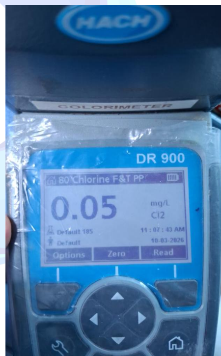
Free chlorine chiller B 0,05 ppm
